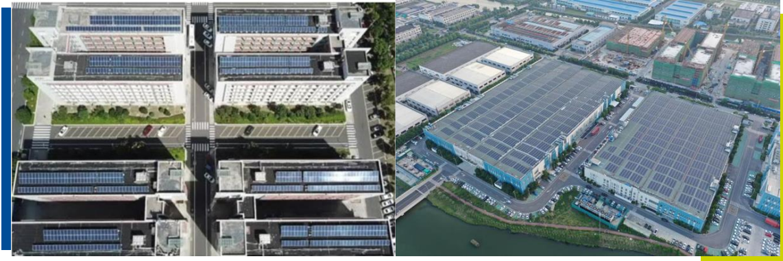
Lanto Electronic Limited Photovoltaic Project
